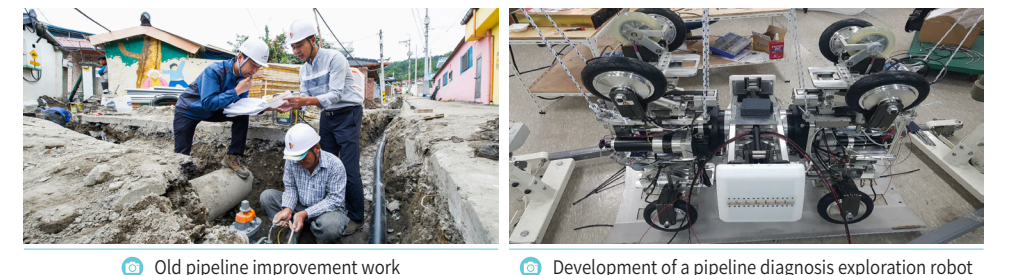
Old pipeline improvement work
