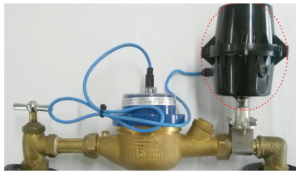
12 Leakage monitoring sensor
