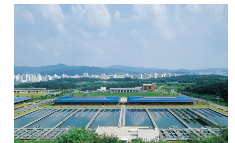
Seongnam Water Purification Plant
