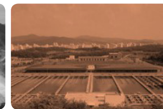
Construction of large area industrial water supply systems in the metropolitan areas of Ilsan and Ulsan, etc.
