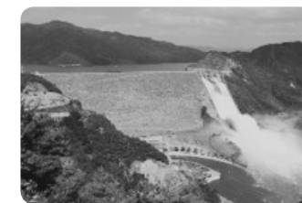
Construction of Soyanggang, Andong and Daecheong Dams
