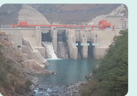
<Patrind Hydropower Plant>
