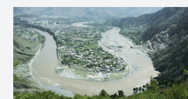
[Pakistan] Patrind Hydroelectric Power Generation Project
