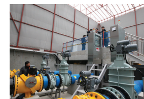
Raceway of Boryeong Dam
