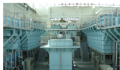
Test plant in the Waterworks and Sewerage Research & Education Center
