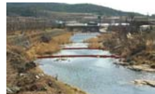
Installation of turbidity and pollution preventing blocks
