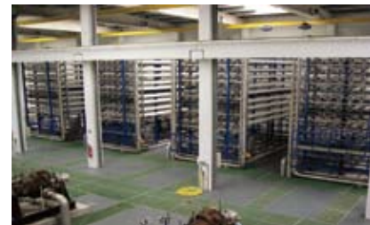
In Water & Sewage Research and Education Center Treatment Demonstration Plant
