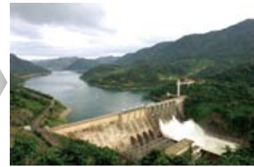
Simultaneous accomplishment of zero flood damage and securing the largest reserve volume in history
