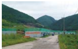
Dustproof Cover Installation
