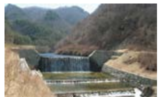
Erosion control dam
