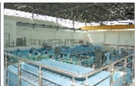
Water & Sewage Treatment Demonstration Plant
