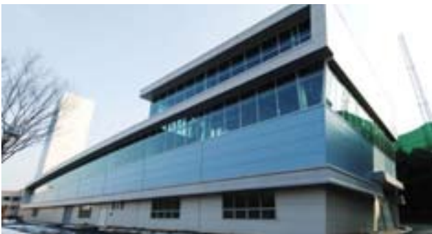
Flow meter calibration center
