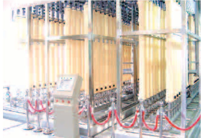
| Screen filtration purification facility in Siheung purification plant |
