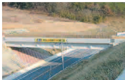
| Overpass-type Wildlife Corridor at the Pyung-lim dam |
