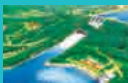
Construction of Environmentally-Friendly Eco-Dam (Hwabuk Dam)
