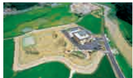
Jinan Sewage Treatment Plant
