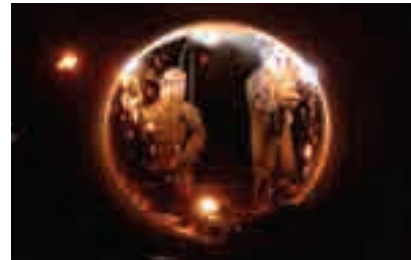
Welding work being performed inside water supply pipes
