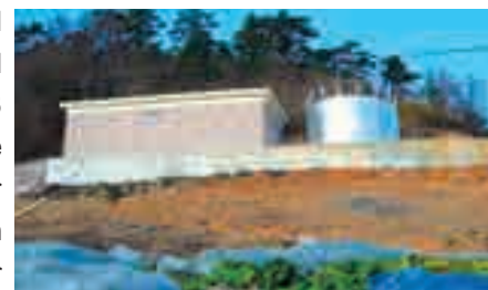
Seawater Desalination Plant in Jabong Island, Yeosu
