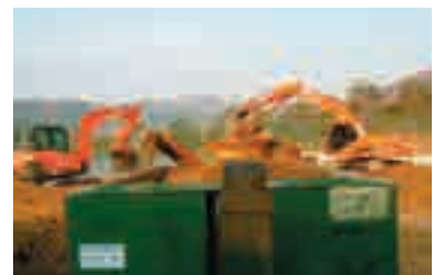
Producing wood chips from forest tree waste
