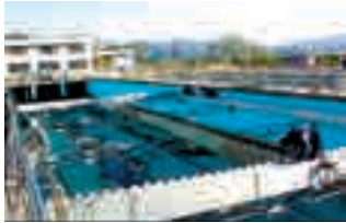
Renovated settling pond
