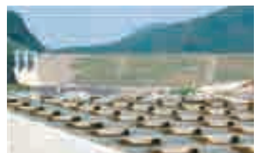
Fish-way downstream of a dam
