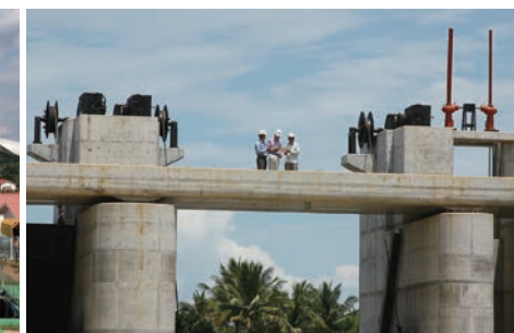
Cambodia Krang Ponley Water Resources Development Project
