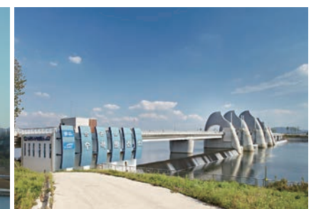
Seungchon Weir Hydropower Plant
