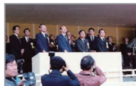
Dec. 02, 1980 Completed the construction of Daecheong Multi-purpose Dam
