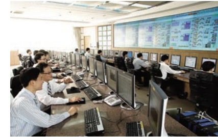
The Metropolitan Integrated Waterworks Operation Center
