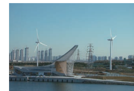
Ara Waterway Wind Power Plant
