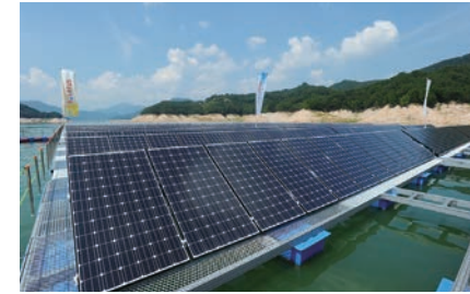
Floating photovoltaic power plant on Hapcheon dam
