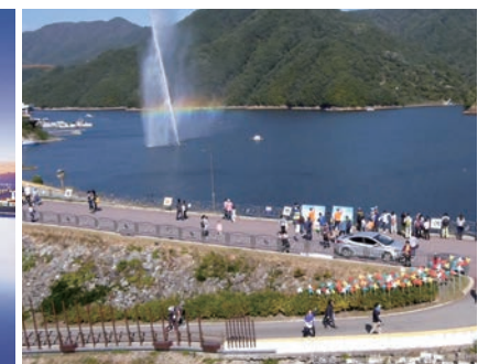
Soyanggang Multi-purpose Dam
