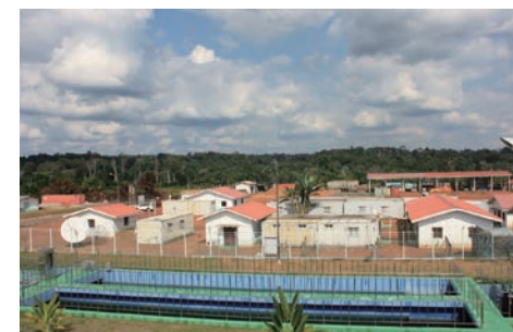
Equatorial Guinea Water Treatment Plant
