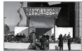
Nov. 25, 1972 Commenced construction of Soyanggang Multi-purpose Dam
