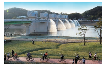
Construction of a waterfront bike trail
