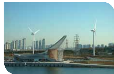
Gyeongin wind power plant
