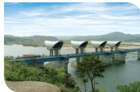
Baekjae barrage small hydroelectric power plant
