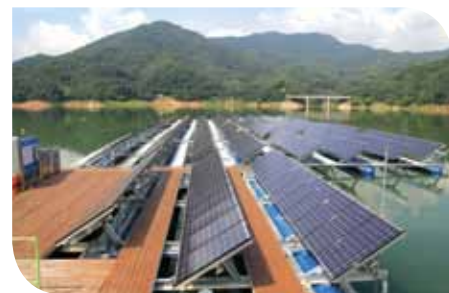
Floating photovoltaic power plant on Hapcheon dam
