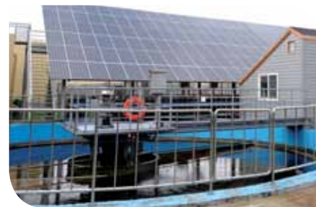
Boenn sewage treatment plant
