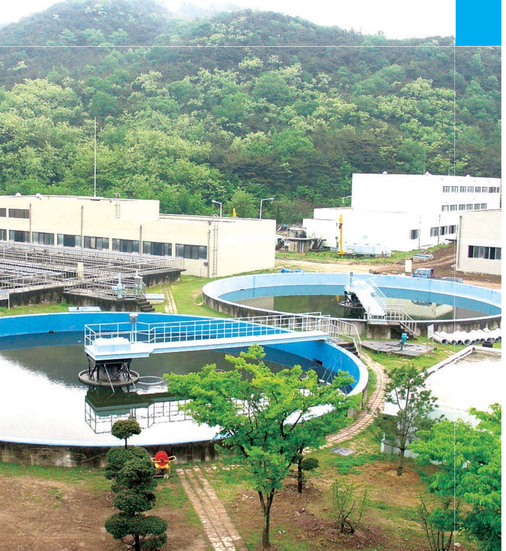
Waegwan sewage treatment plant
