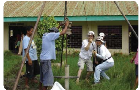
Build water supply facilities in Laos
