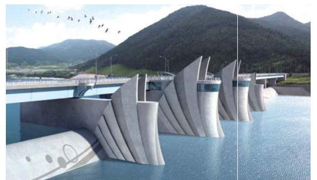
Aerial view of four-river small hydroelectric power plants
