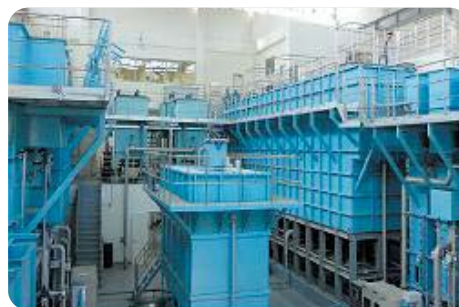
Water supply and drainage education center
