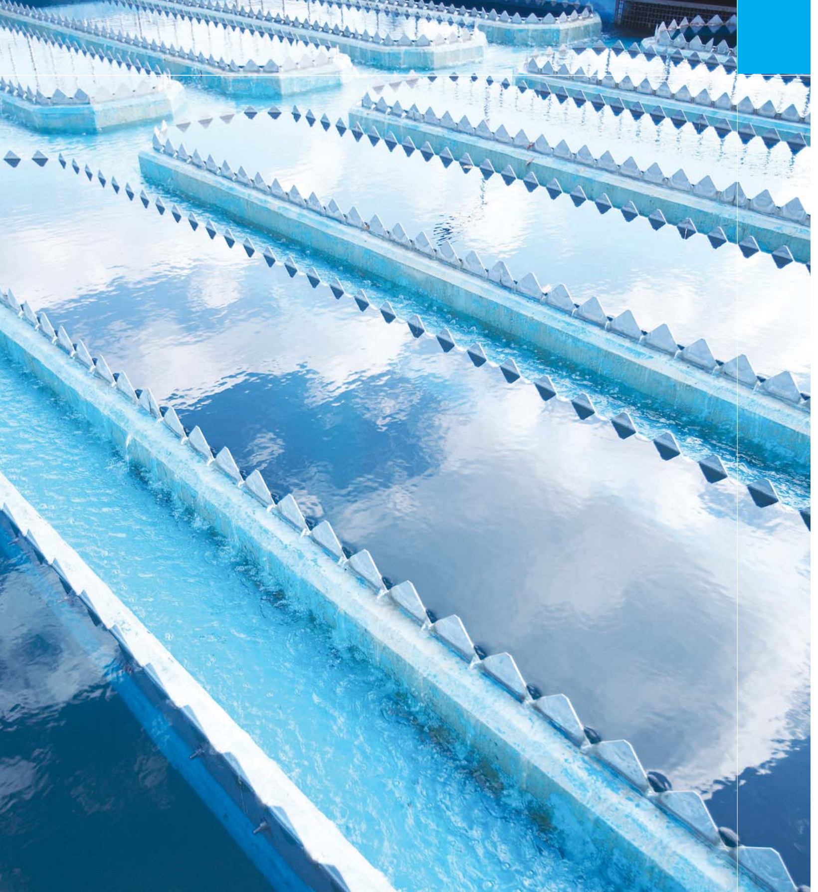
Front view of water purification facilities
