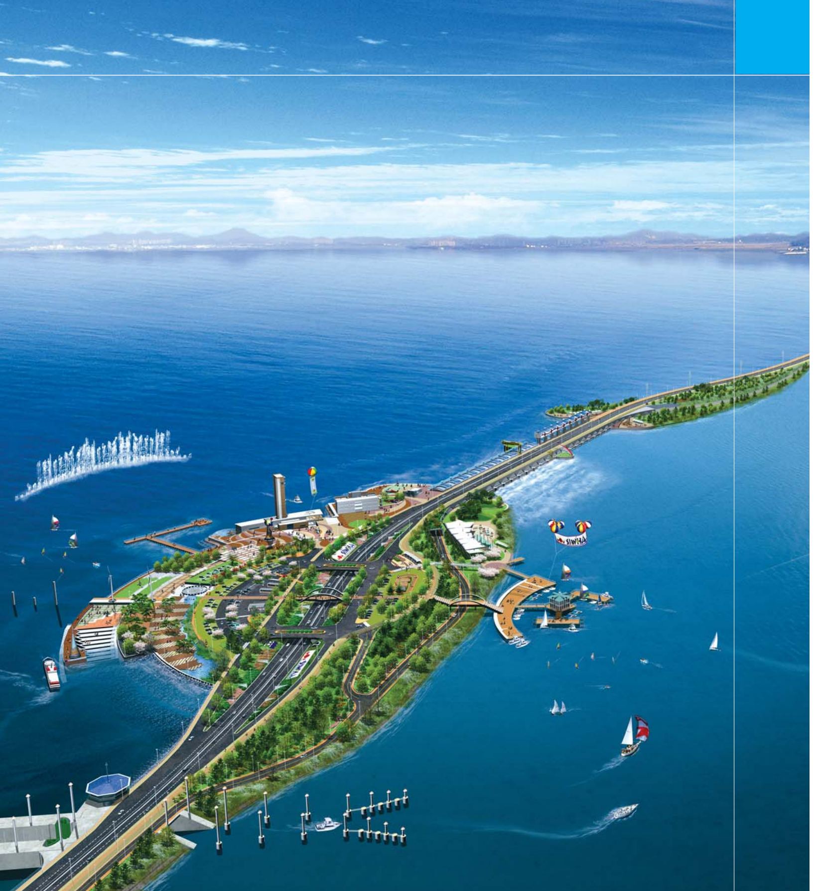
Aerial view of Sihwa tidal power plant
