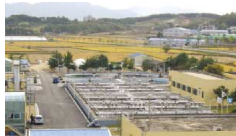
Boeun Wastewater Treatment Facility
